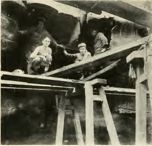
HOLE IN HULL OF "MOUNT VERNON" CAUSED BY TORPEDO
