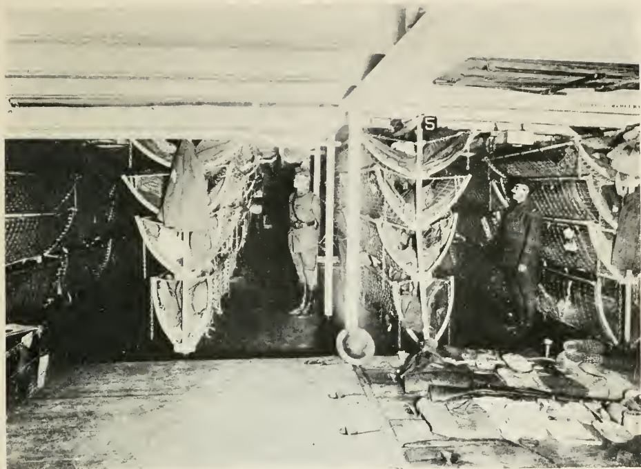
BUNKS TRICED UP FOR INSPECTION
