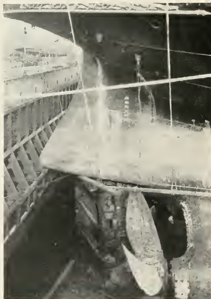
"AGAMEMNON," EX-KAISER WILHELM II. POINT OF STERN PROJECTING BETWEEN BRACES OF CAISSON, RUDDER SWING 60° TO PORT TO CLEAR CAISSON
