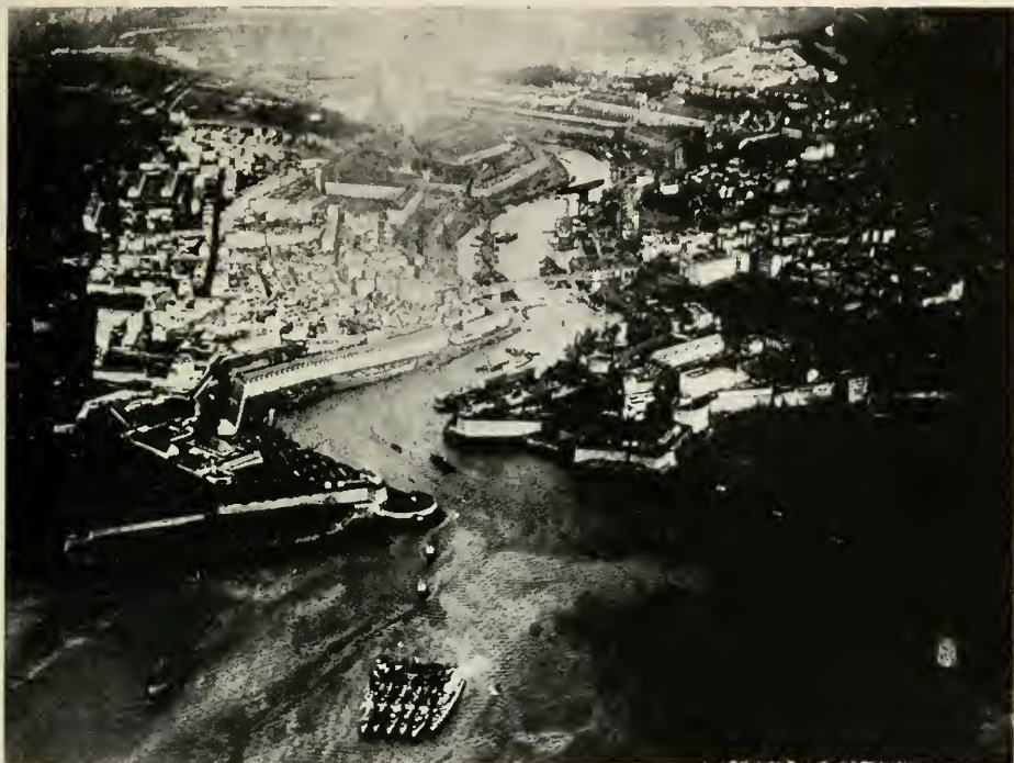
BIRD'S-EYE VIEW OF THE HARBOR OF BREST
