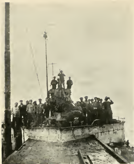
THE U. K.-152 ON WATCH FOR ALLIED SHIP- PING. PHOTOGRAPH TAKEN BY A MEMBER OF THE GERMAN CREW ON OCTOBER 12, 1918. NOTE THE LOOKOUT ON FOLDING MAST
